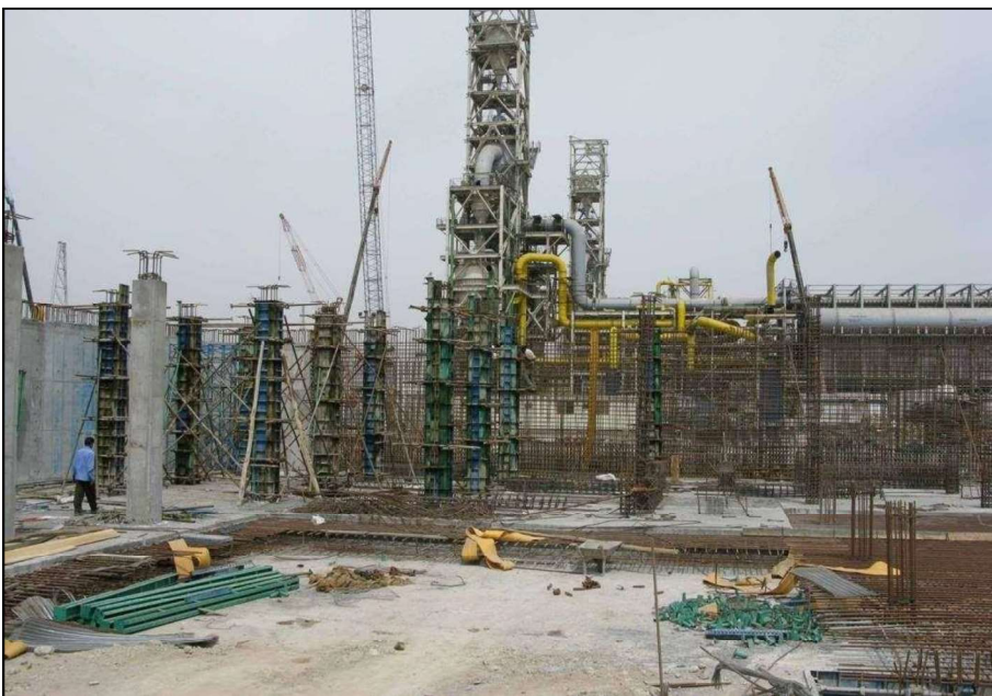
SMS DEMAG-INNSE - Mobarakeh steel complex (Iran)
