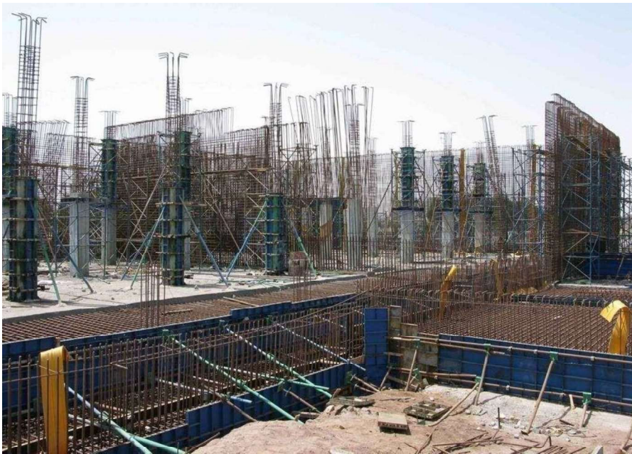
SMS DEMAG-INNSE - Mobarakeh steel complex (Iran)
